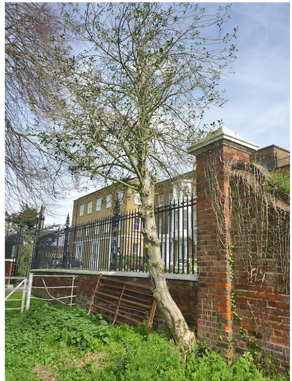
28. Holly: Extensive damage at base. Remove.
