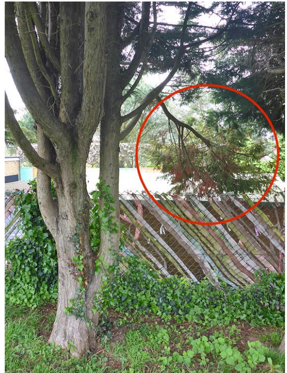
4. Leyland cypress: Remove branch collapsing onto shed roof.
