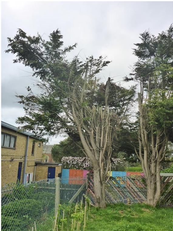
7. Leyland cypress: Remove. N.B. whole row is in poor condition - consider removal and replacement planting.
