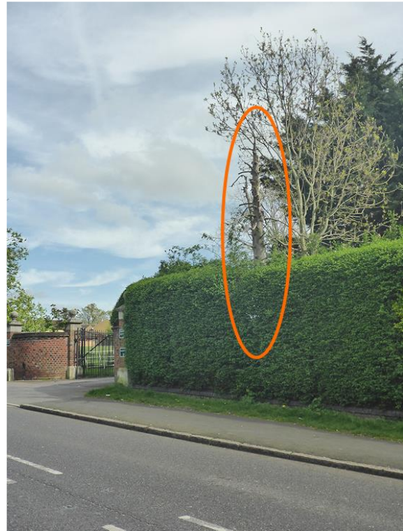
18. Dead: Within falling distance of road. Remove.
